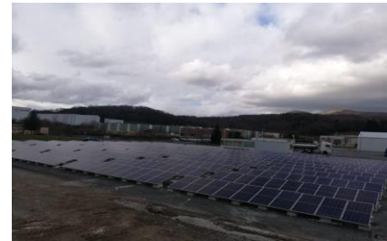
240 kWp (Lecumberri; Navarra)
